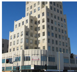
Typical pre-1978 "soft-story" non-ductile concrete structures
