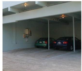
Typical pre-1978 "soft-story" wood frame buildings in Los Angeles
